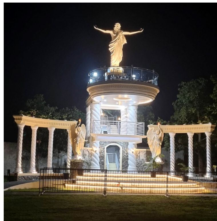
GRATEFUL|| Fr. Wilmer Joseph Tria also thanked Architect Severo, a creative and environmentally-conscious builder who personally supervised the design, construction and eventually the erection of the Easter Angel Tower. Severo was Tria’s former classmate at the Naga Parochial School and at the Holy Rosary Minor Seminary.
